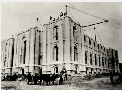
Building the Mormon Temple in Salt Lake City
